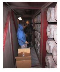
Inside the air intake filter housing for gas turbines
