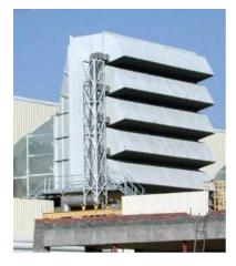
Air intake filter housing for gas turbines
