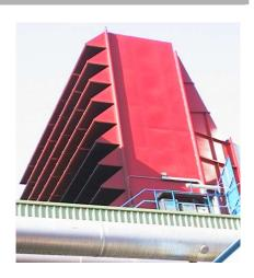
Air intake filter housing for gas turbines
